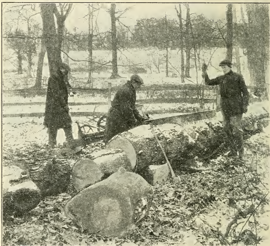
Fig. 127. A motor driven drag saw in action
